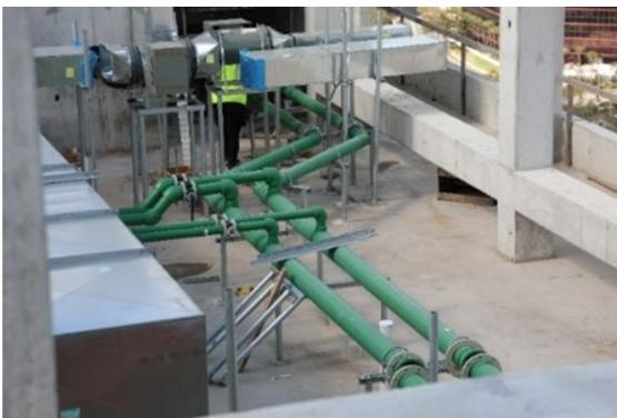
The HVAC mechanicals for the project include a hybrid air-and-water system involving condenser-chilled water from a rooftop cooling tower pumped
