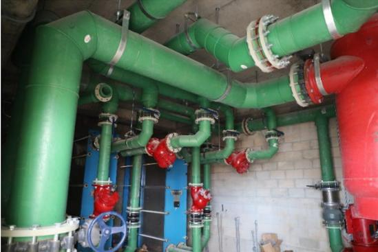
The 800 feet of PP-RCT pipe supplies and returns water to the rooftop cooling tower. Joining sections and fabricating the various angles was done by heat fusing the sections together. This eliminated open-flame welding required for carbon steel and iron pipe, plus increased safety and sped-up the work, especially in tight spaces.
